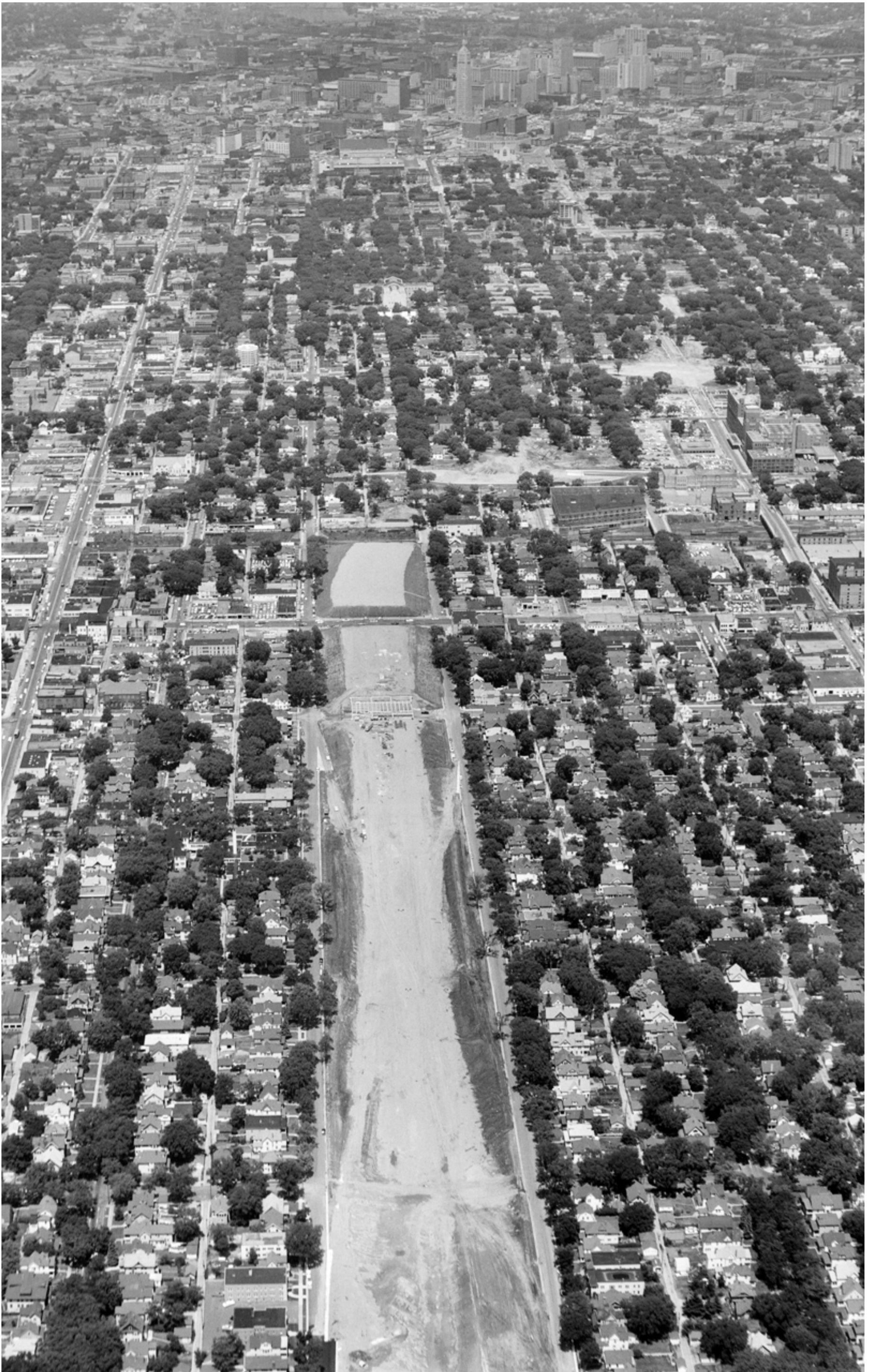
Image 3. An estimated 24,000 people lost their homes, and an unknown number of businesses were affected, as result of freeway construction in Minneapolis. Photo of I-35W under construction circa 1963, courtesy of Minnesota Historical Society.
