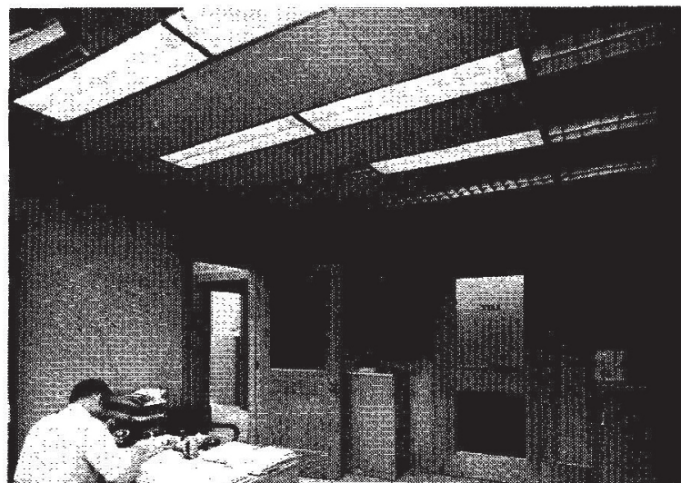
Figure 6. A portion of the office with the experimental control systems in use. The microcomputer and controls are in the cabinet at the left side of the door.
