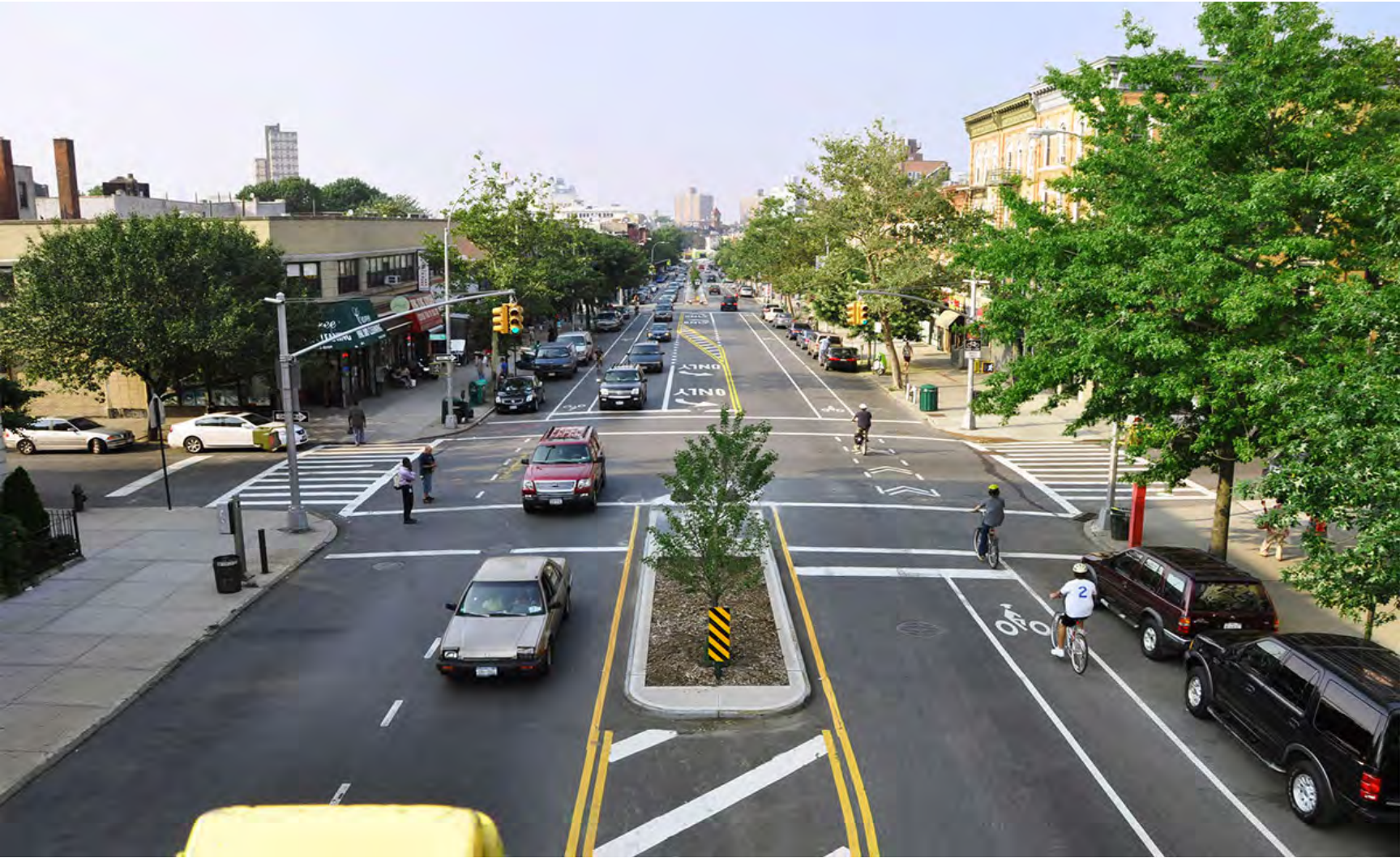
Figure 49: Clearly marked roadways help promote safe multimodal roadway design. Brooklyn NY
