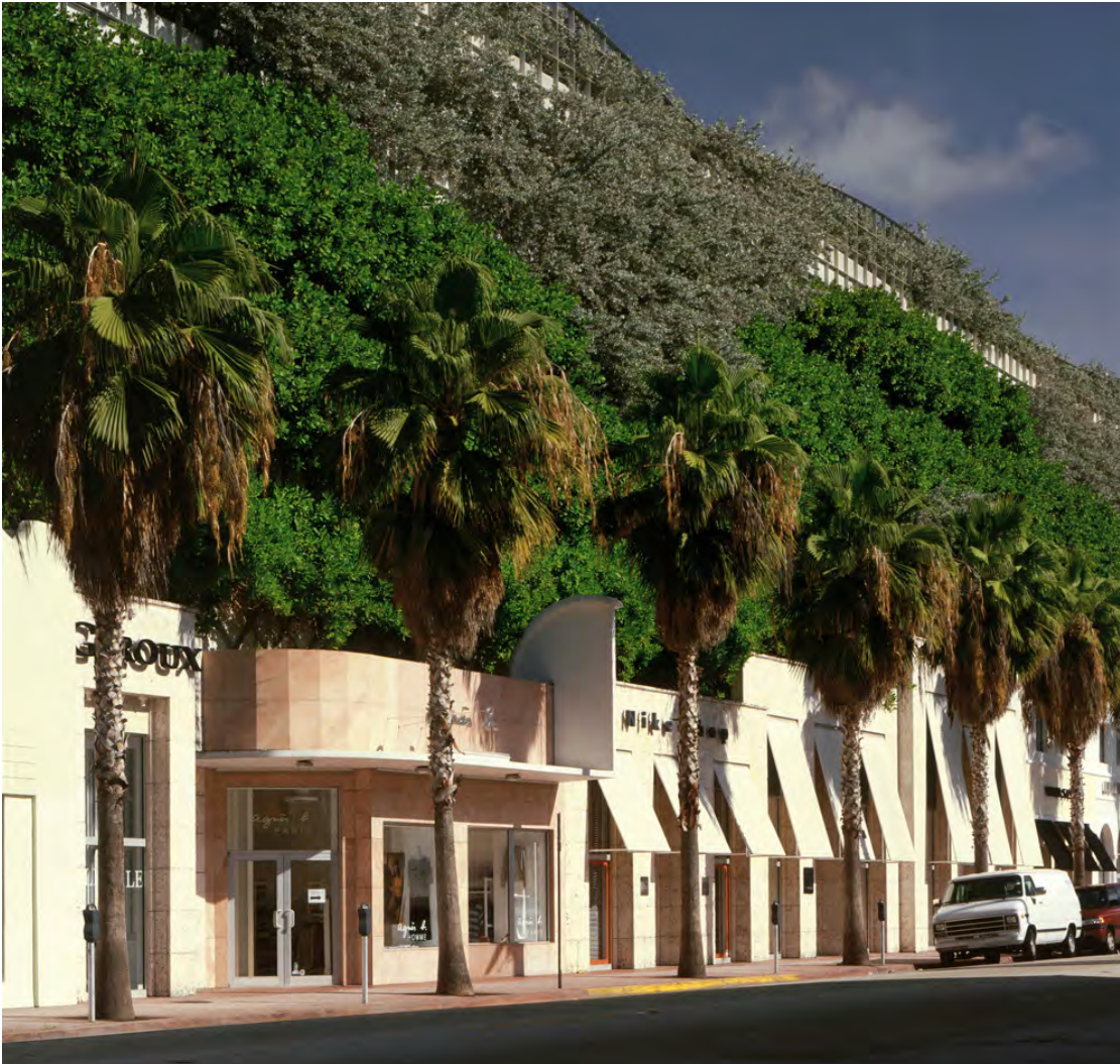
Figure 153: Parking structure with shops on first level and green wall covering parking levels above positively impacts the pedestrian environment. Miami Beach, FL
