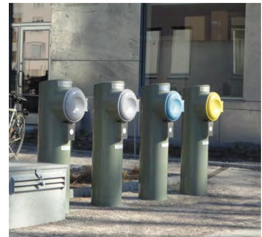
Figure 149: Centralized waste management systems eliminate trash collection vehicles and can separate waste for energy generation. Stockholm, Sweden
