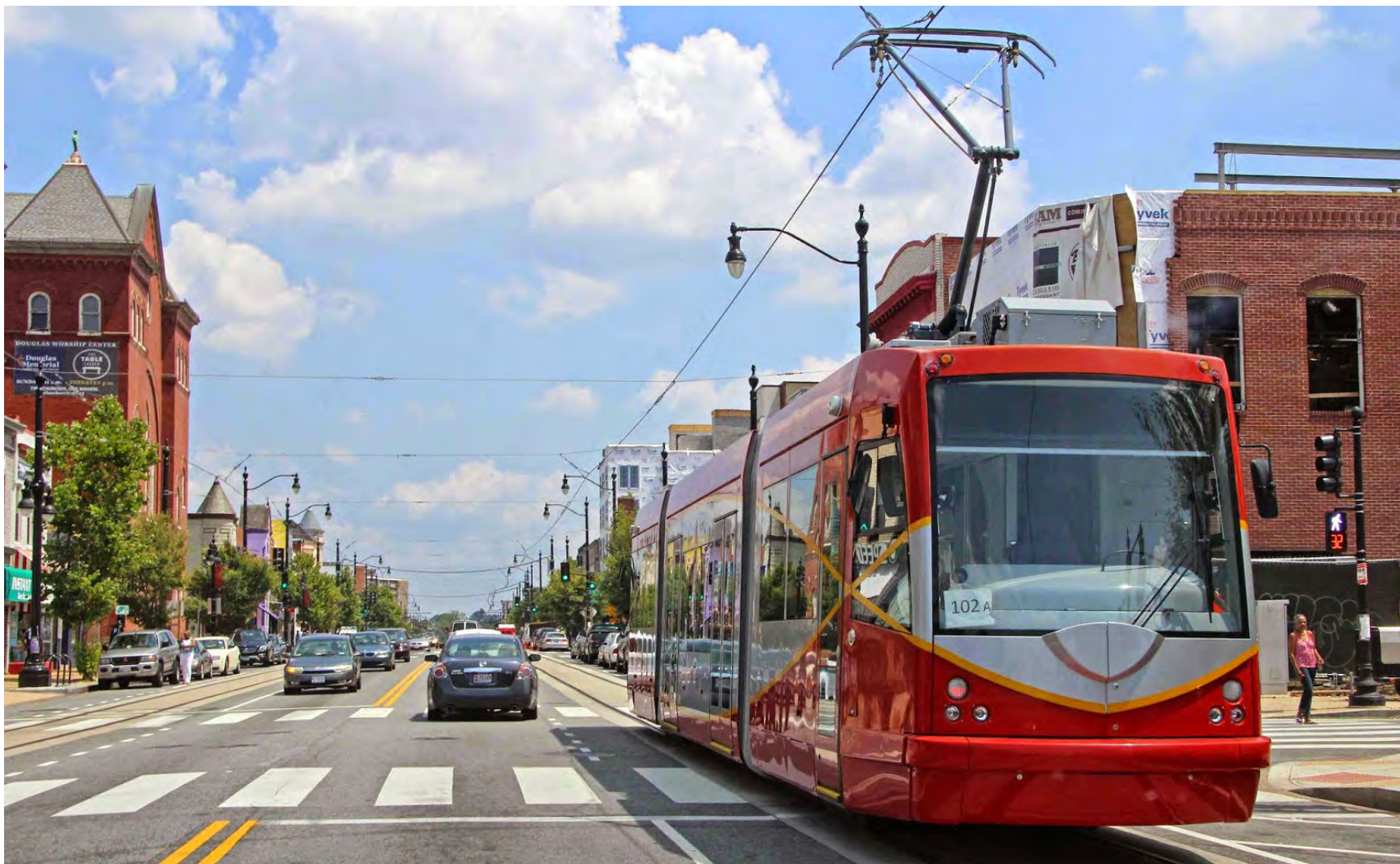
Figure 45: Modern streetcars in dedicated guideways share the street with cars and parallel parking. Washington DC
