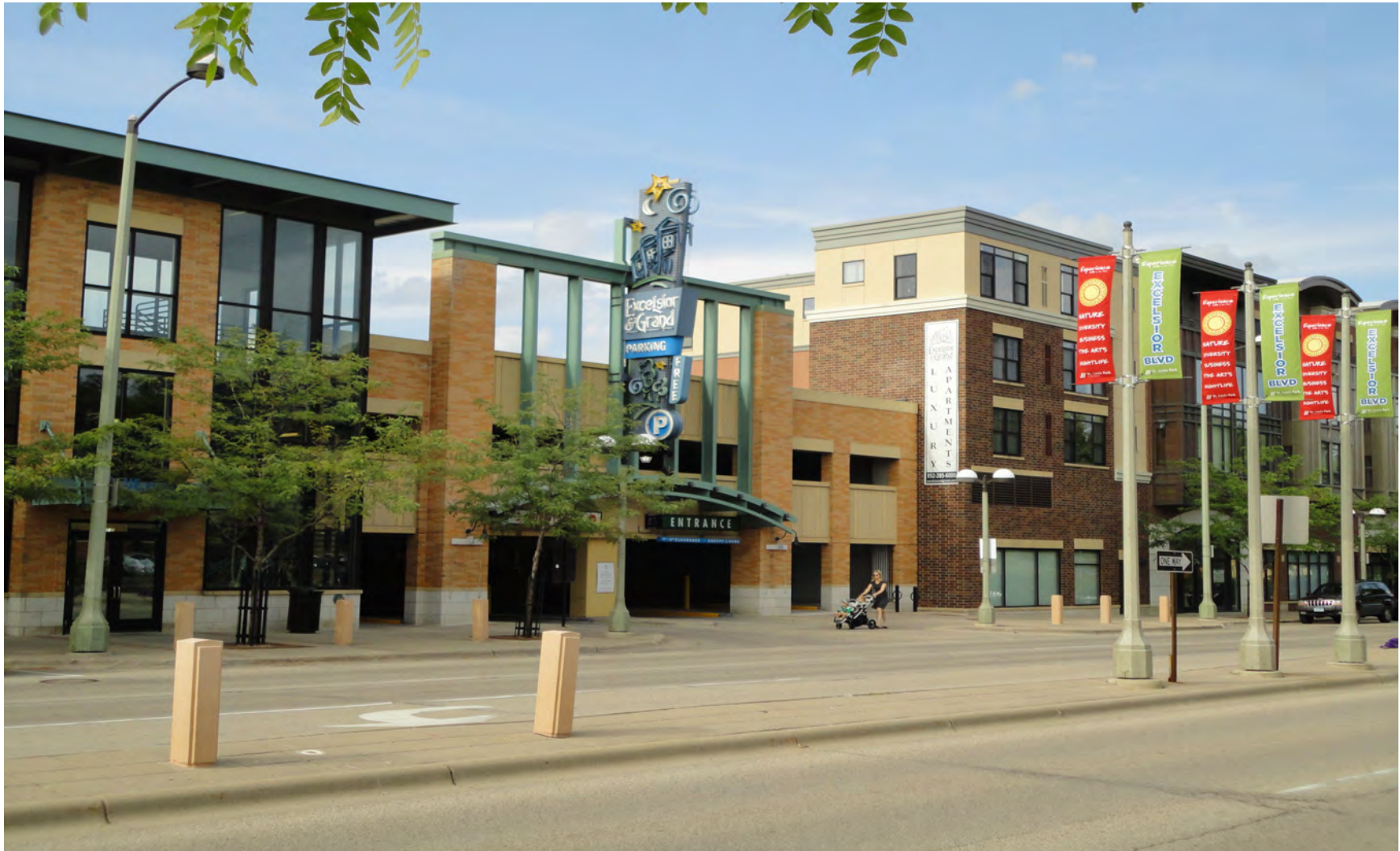
Figure 17: District parking is seamlessly integrated into the design and placed in the center of the block. St. Louis Park MN
