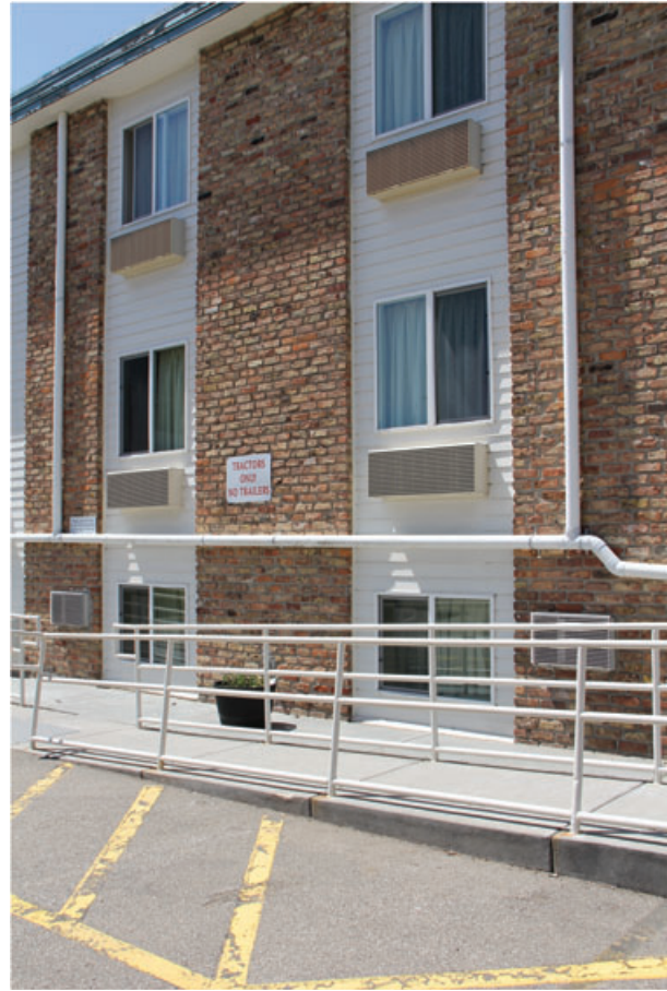
Figure 8. Ground floor rooms and windows are conducive to direct room access.
